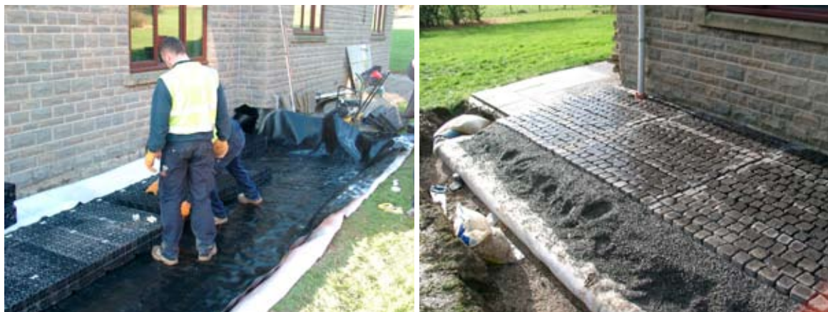
Installation of a rainwater harvester system below a permeable concrete block surface
